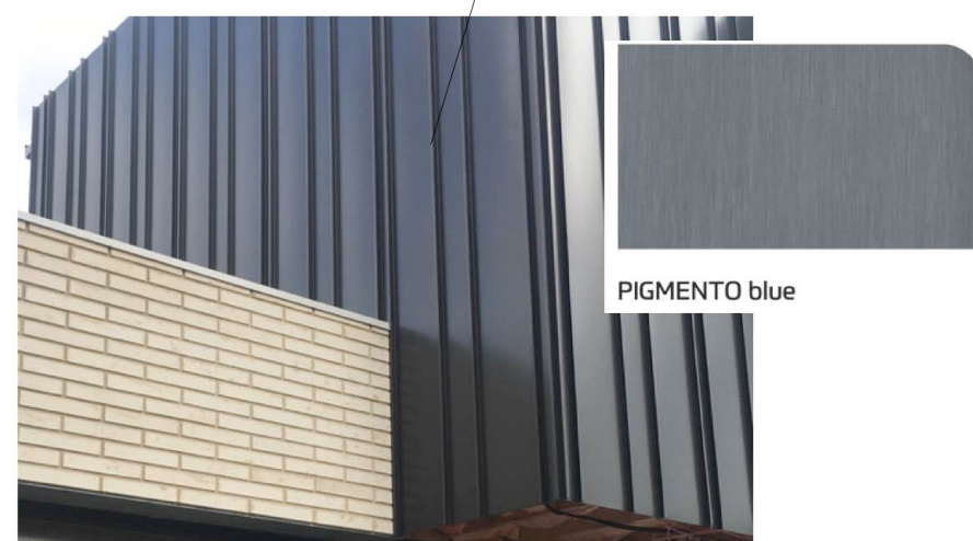
Walls - Standing seam Metal (Blue - various widths)
